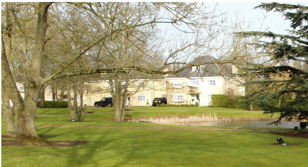
View across New Hall parkland of the new Paddocks housing.
