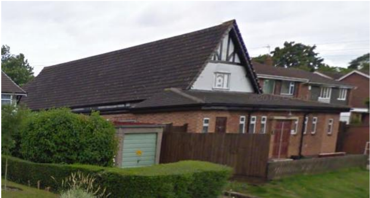
The Memorial Hall, Anstey Road, showing the unsympathetic design of the front extension.
