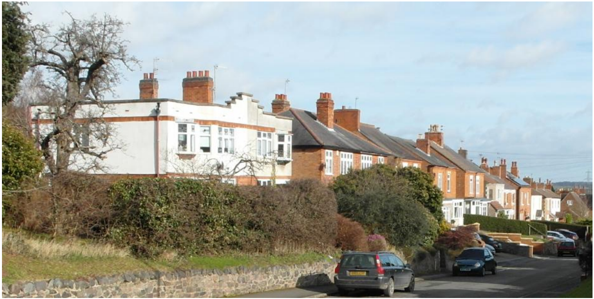
8 – 38 Narrow Lane – view from west.
