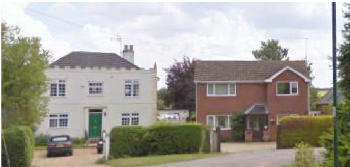
Inappropriate design of C20th house adjacent to The Standings.
