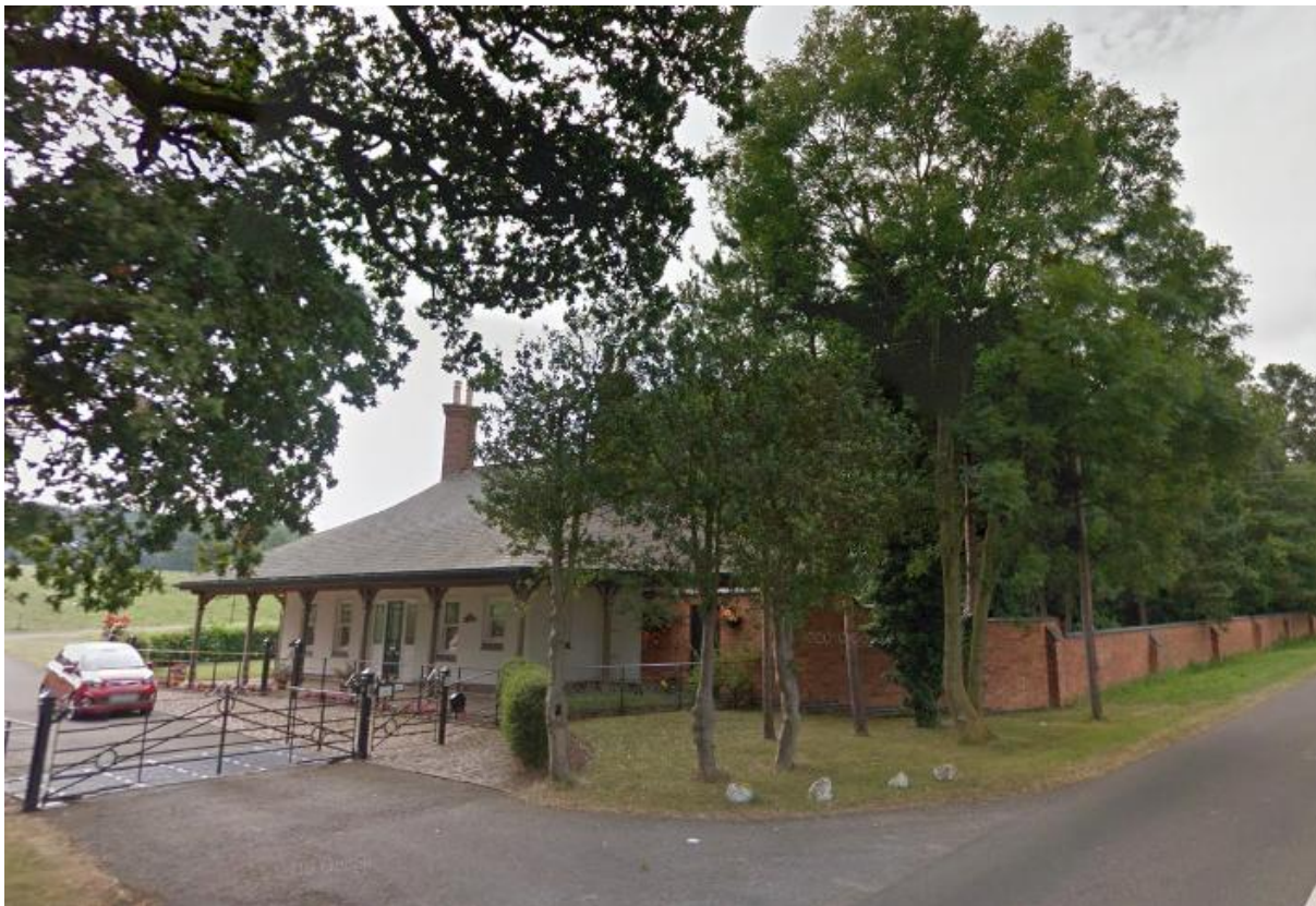
Queniborough Road entrance lodge to Barkby Hall is shown on 1884 OS map.
