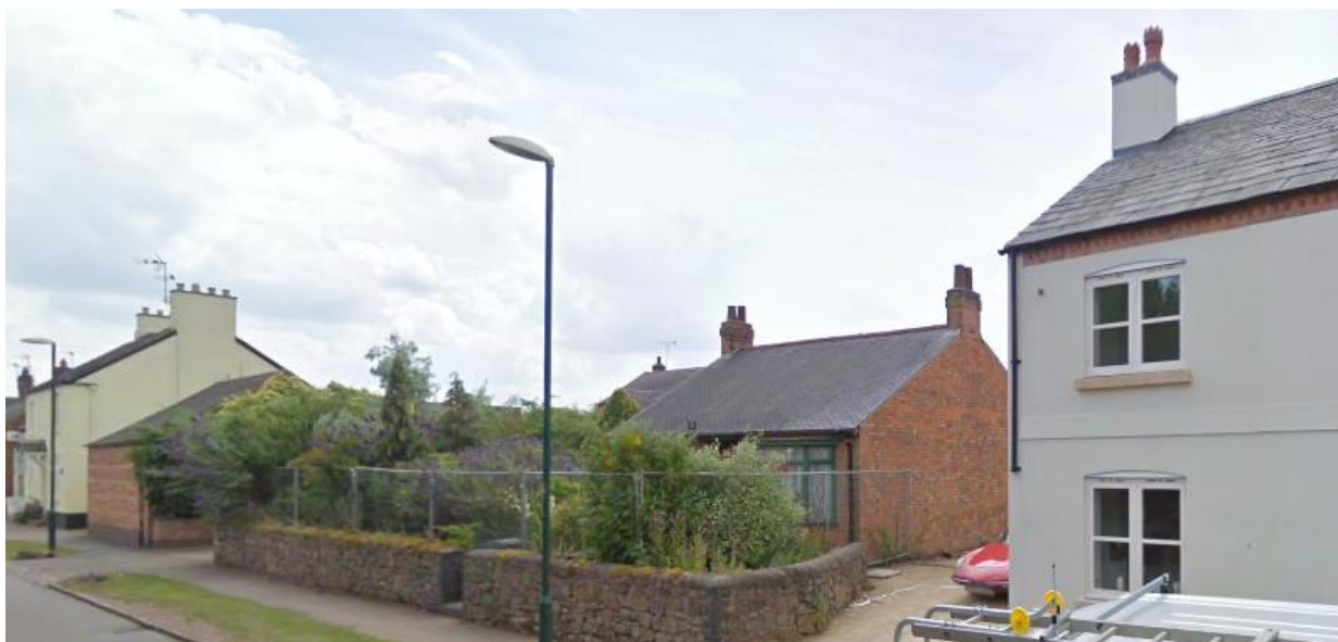
Unfortunate gap in traditional village frontage created by set-back, scale, form and design of infill development
