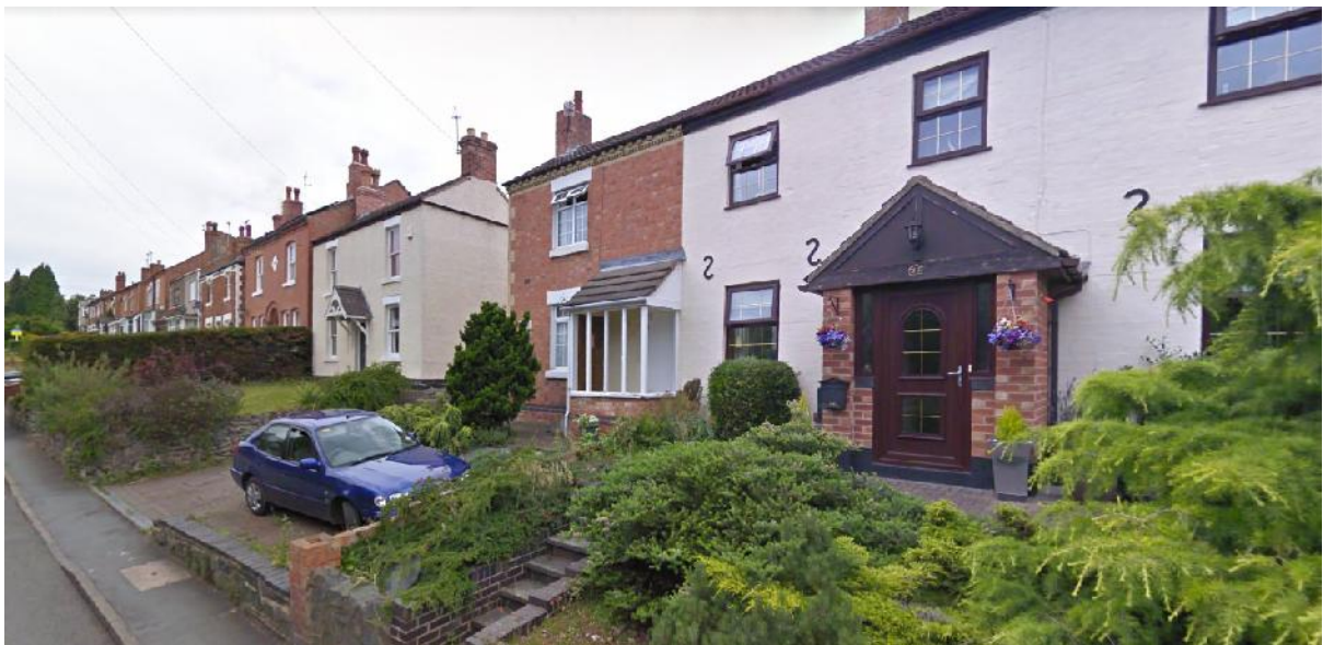
Add no's. 8 – 38 Narrow Lane, an attractive streetscape of Victorian terraces, most shown on the 1883 OS map – view from east.
