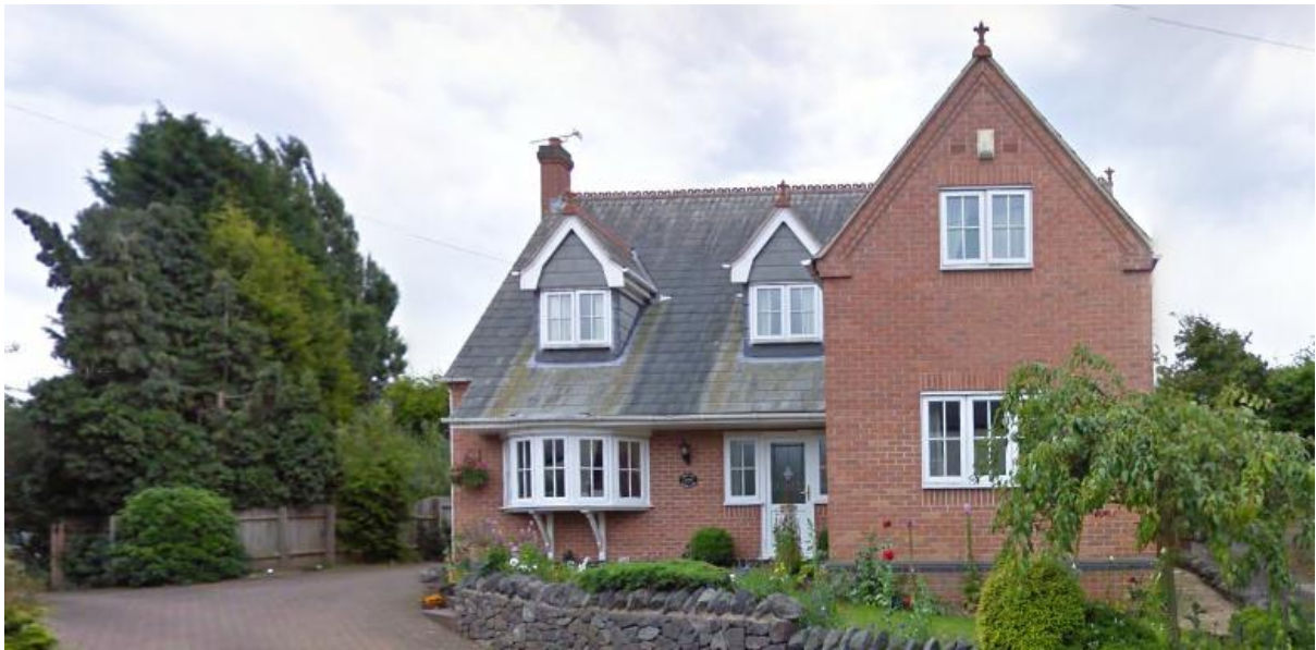
Omit: recently built 31 Narrow Lane – southside.
